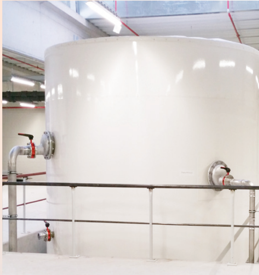
Our 79,000 l tank is 6.8 m high and covers two floors
