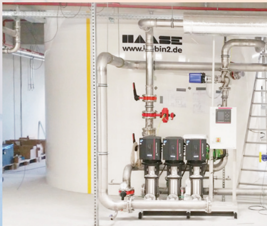
Our 79,000 l tank is 6.8 m high and covers two floors
