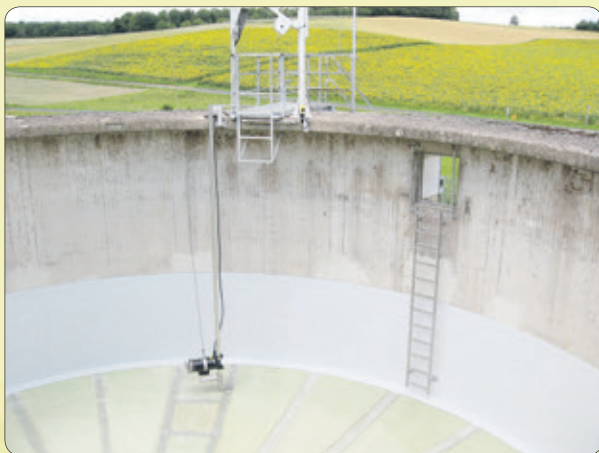
Due to the dimpled underside of the GRP laminate, possible irregularities in the substrate are evened out. At the request of the customer, a protective paint can be applied.
