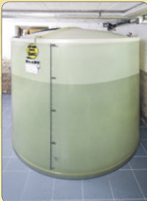
Due to the transparent tank wall, the fluid level can be read at all times without problem.
