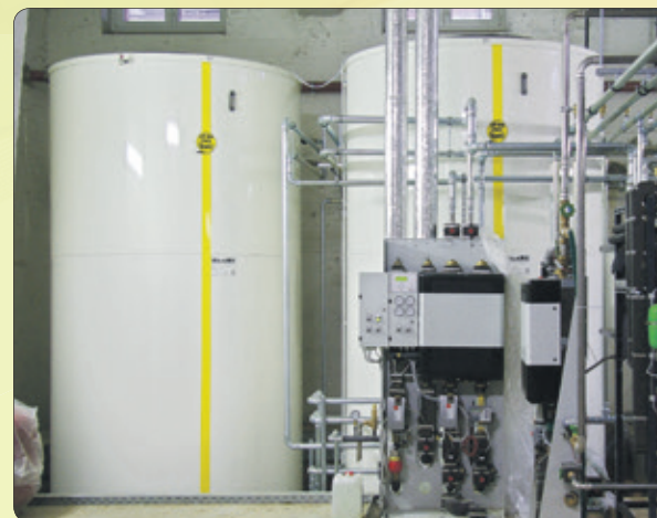
The charging and discharging can be via flange, internal heat exchanger or stratification system.
